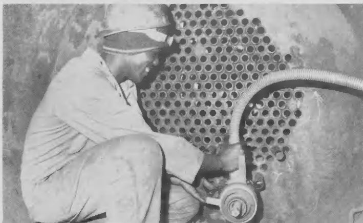
With the tube puller machine a larger amount of tubes were pulled in less time .....
